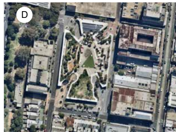
After: 2 level basement car park with rooftop park and community amenities at grade
