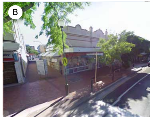
Before: Woodville Lane and council purchased properties
