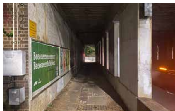
Uninviting public footpath on Raw Square underpass
