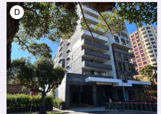
Churchill Ave and Albert Rd height transitions
