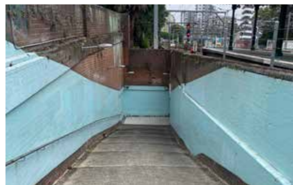
Uninviting pedestrian tunnel across railway corridor
