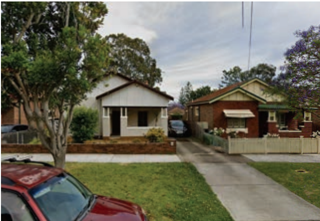
9. Cartwright Avenue, Homebush, looking northwest towards Coleman Avenue
