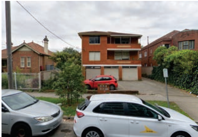
Looking west towards Knight Street
