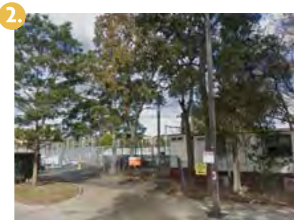
Screenshot of the Homebush Control Centre, as seen from the street facing south. Image from Google Maps.
