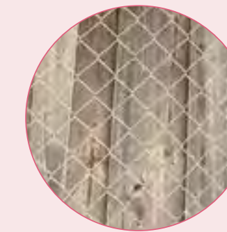
Chain wire fencing
