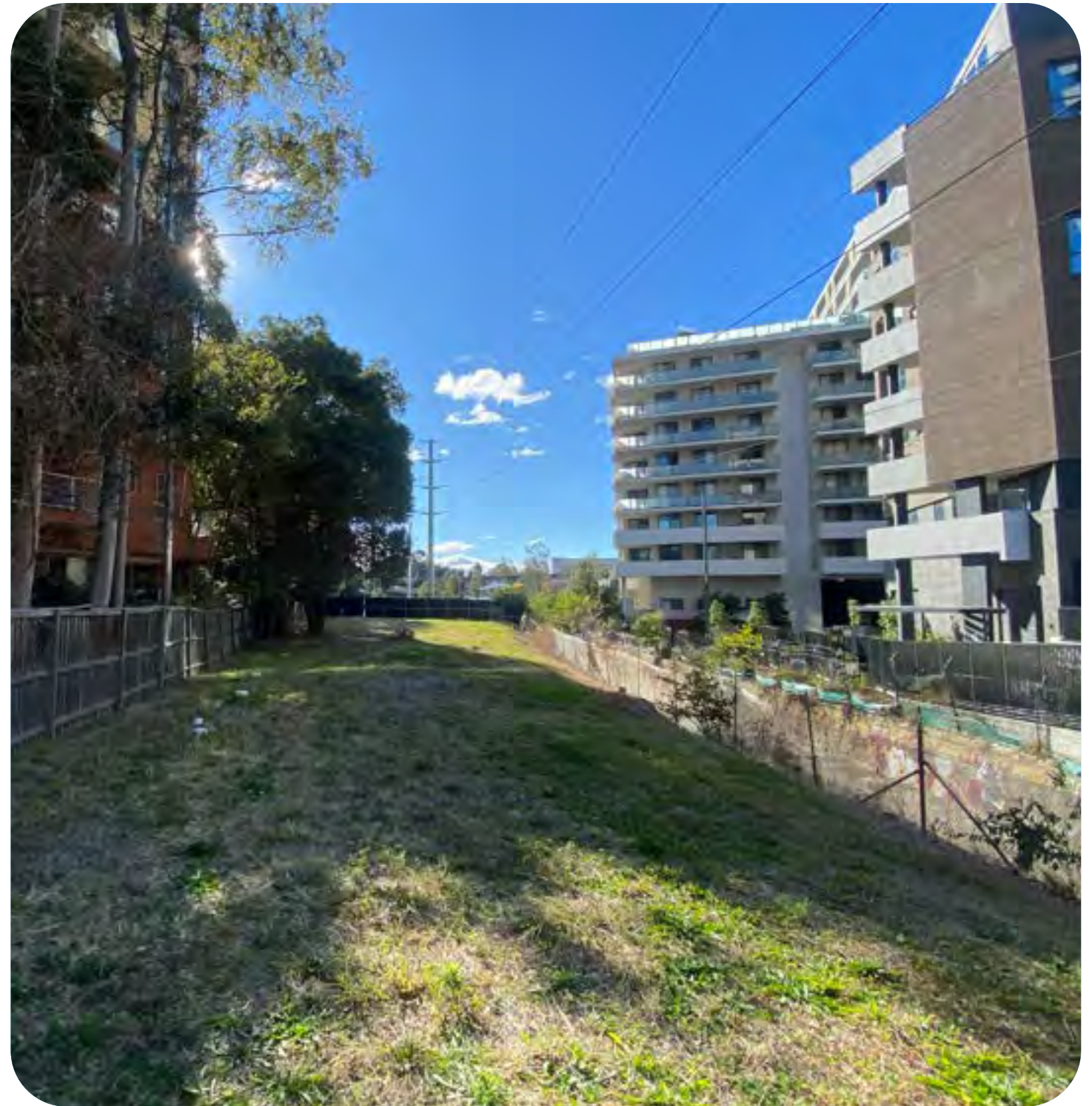
▲ 20A Parramatta Road is a very narrow slice of land with significant steep slopes towards Powells Creek
